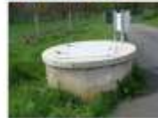
Forages de Ligaine – Talzé (79) : Production SVL
